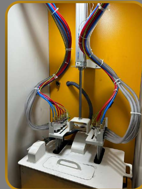
MATECH , PLC controlled Matech brand Paint center equipment; It is a complementary element of paint systems to improve paint quality and rapid color change.
